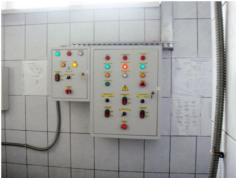
Pilot Production Building – Fire Suppression System
