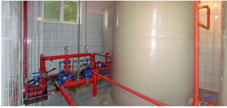
Pilot Production Building – Fire Suppression System
